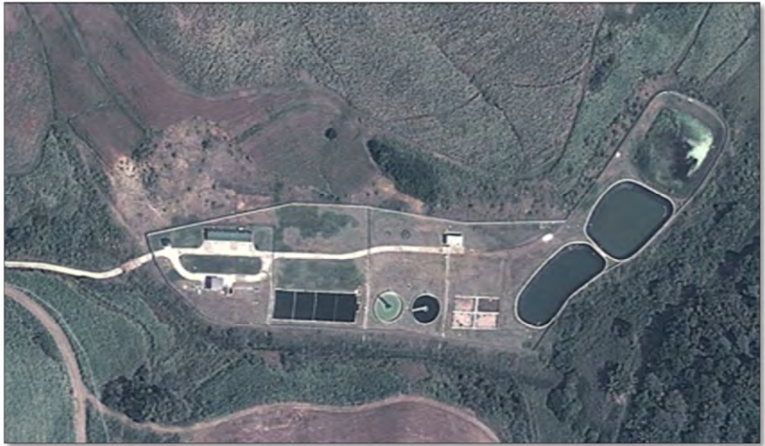
Figure 1 Sheffield Waste Water Treatment Works
